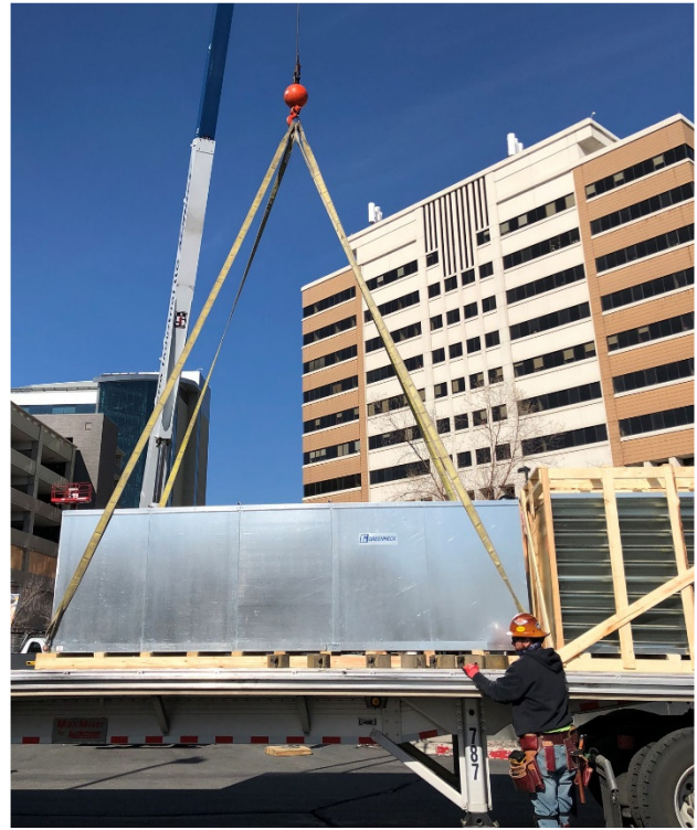
Greenheck Make-Up Air Unit
