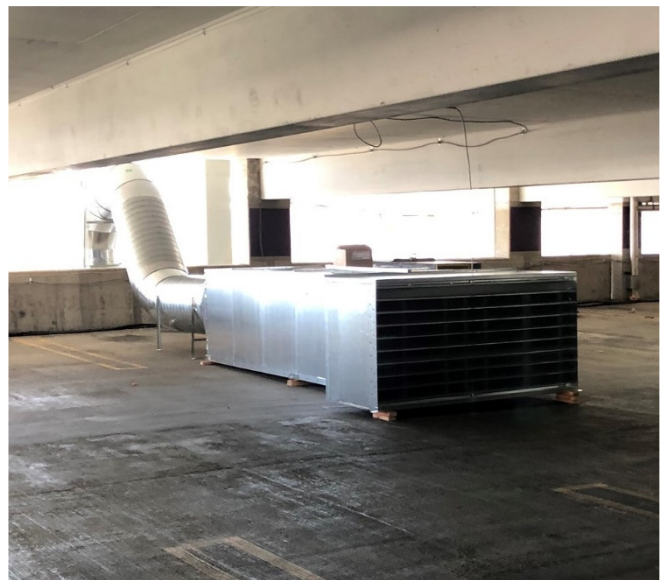
Greenheck Make-Up Air Unit
